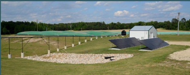
A covered swine waste lagoon biogas project at the Butler Bio Solar Farm, Harnett County, NC. Photo credit: Courtesy of Tom Butler.
