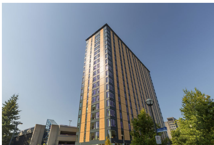
Figure 2. CLT use in Brock Commons Tallwood House in Vancouver, BC ( www.vancouver.housing.ubc.ca ) Source: Brudder, naturallywood.com .
