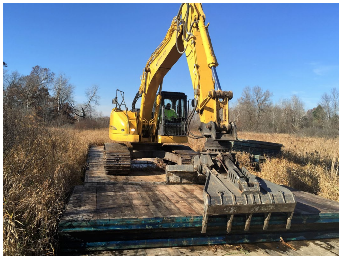
Figure 3. Sterling Lumber CLT matting. Source: SterlingSolutions.com .
